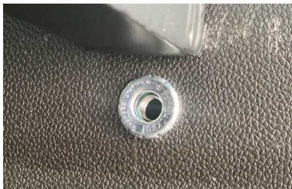
Completed Rivet
